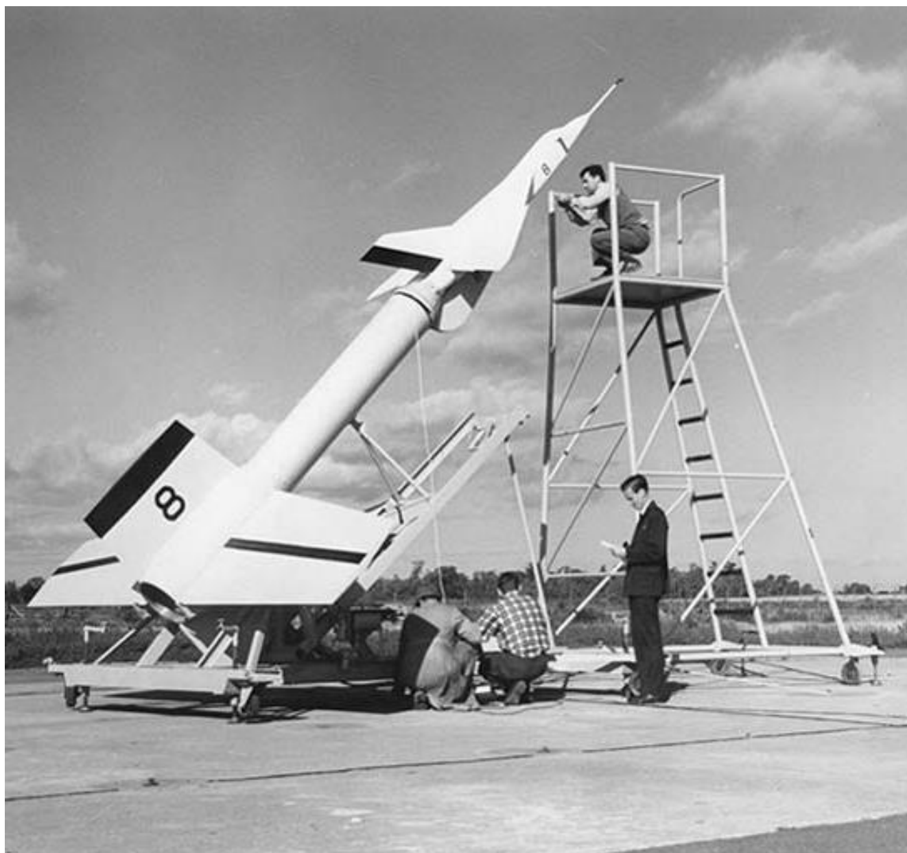
Plate 34: Avro technicians prepare an Avro Arrow test model attached to a Nike booster rocket to fire out over Lake Ontario at Point Petre in the 1950s. Retrieved from: The Orenda Ring | OTTAWA REWIND
