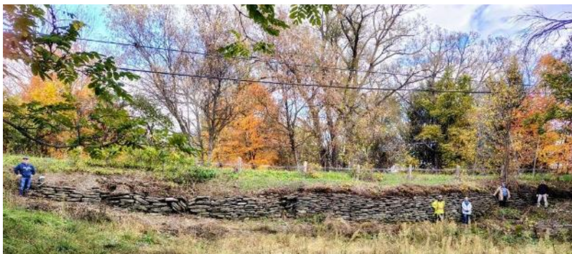
Plate 15: Palen's Bridge, 2025. Photo credit: J.D.Lyons.
