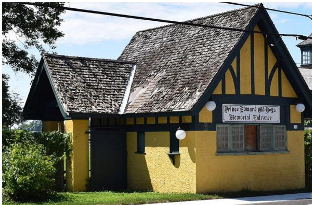
Plate 33: Old Boys Memorial Entrance building. Photo credit: CountyLive, "Old Boys Memorial entrance repairs needed to save building," Retrieved from: Old Boys' Memorial Entrance repairs needed to save building : Prince Edward County News countylive.ca (2025)
