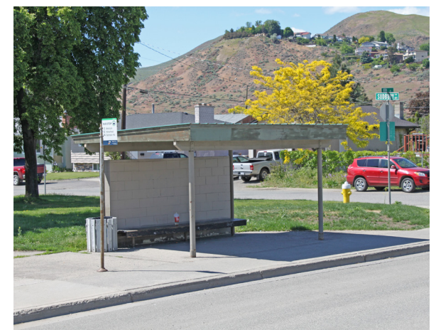
Existing transit stop at 8th Street Park
