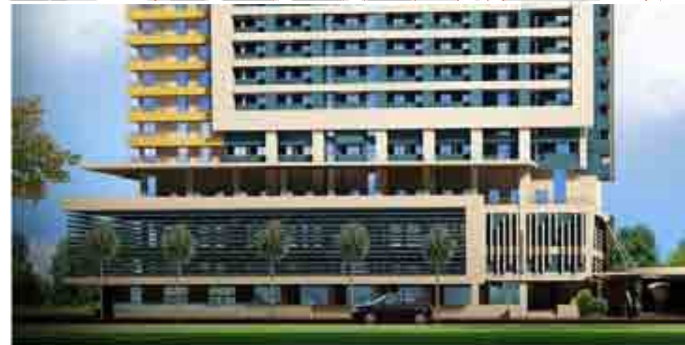
Fig 4.17 Example of upper parking podium
