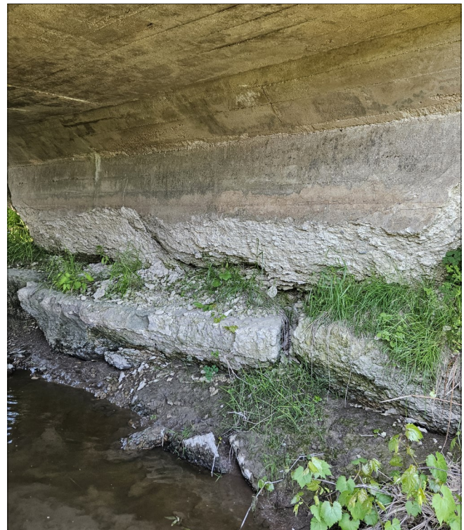
Photo 4 - View of West Footing and Abutment Wall.
