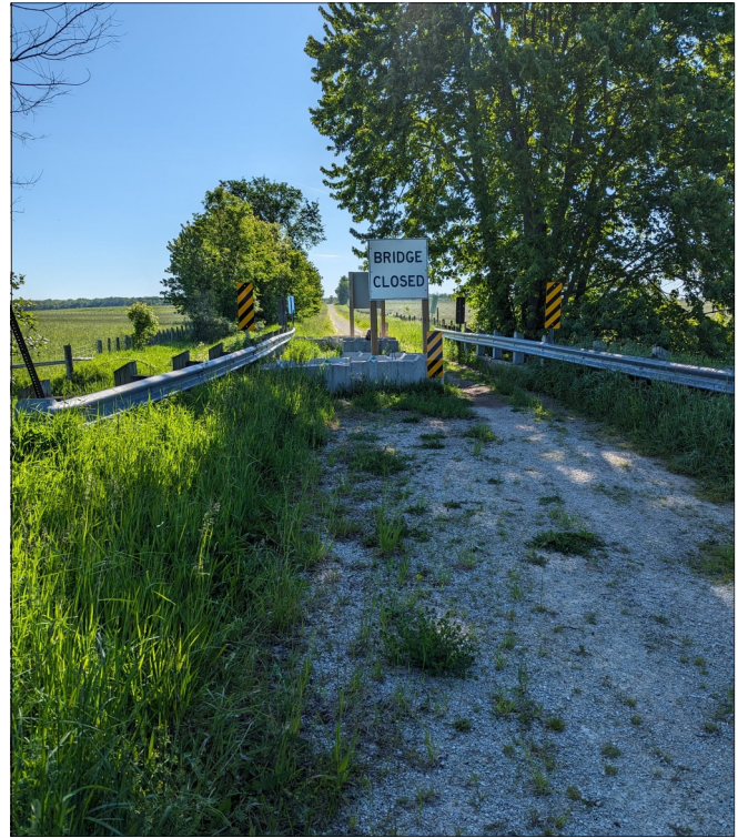
Photo 2 - View of Structure Facing East.
