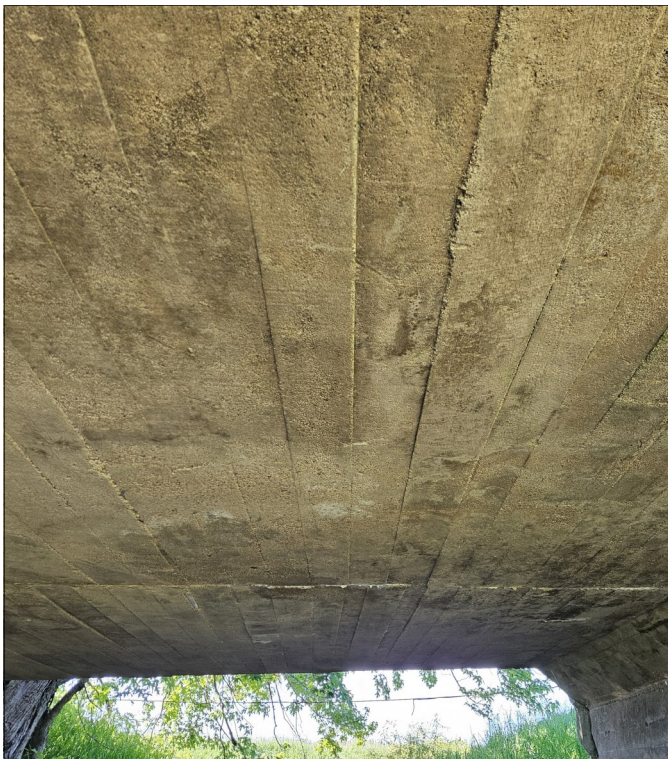
Photo 3 - View of Soffit.
