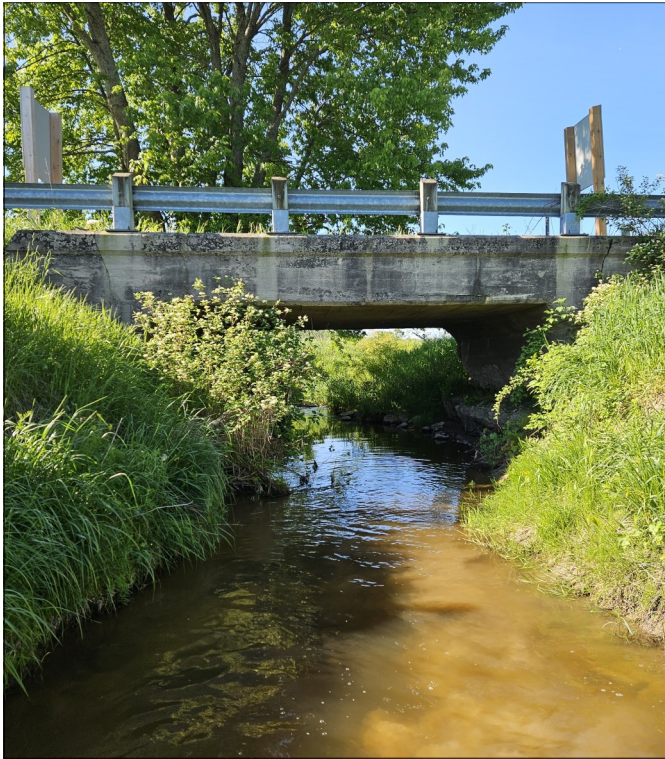
Photo 1 - View of Structure Facing South
