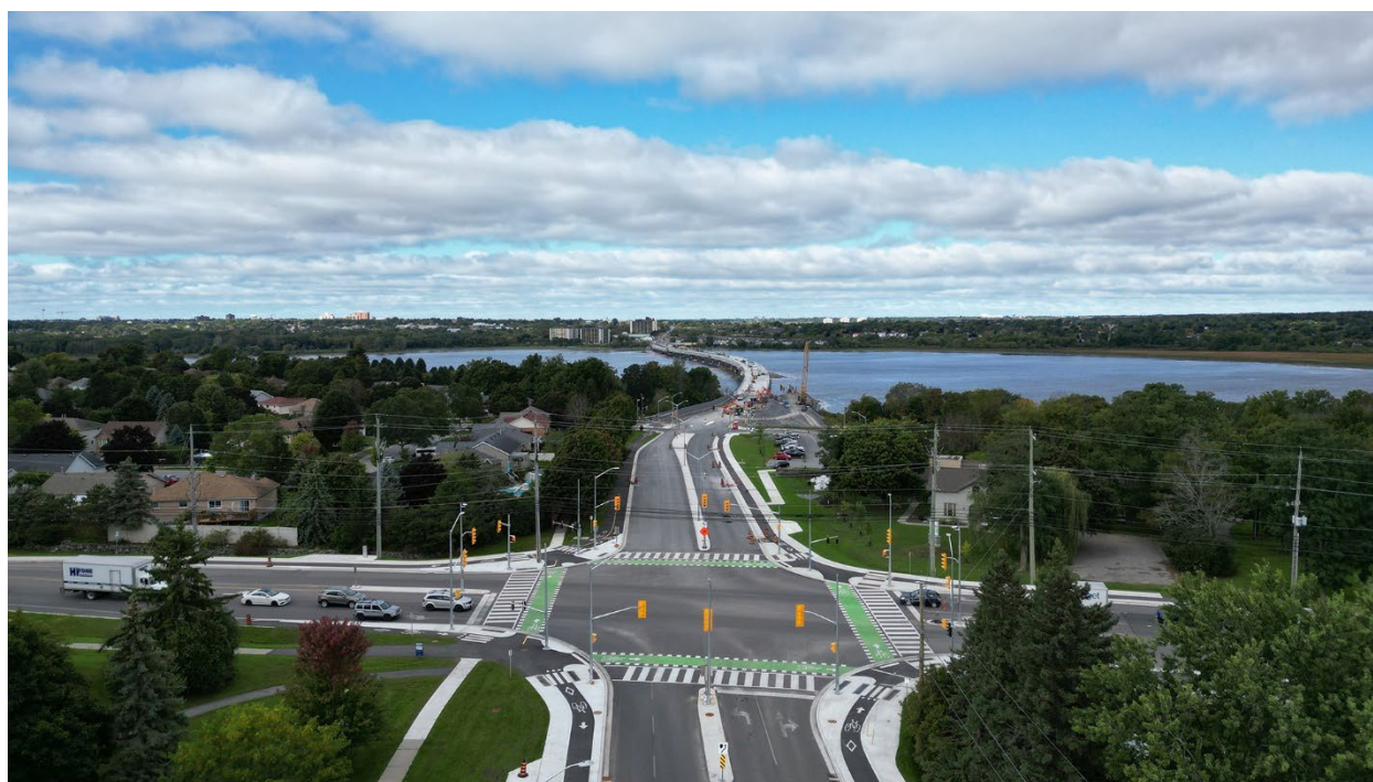
Figure 5.18: Protected Intersection Reconstruction, Kingston (Source: City of Kingston)
