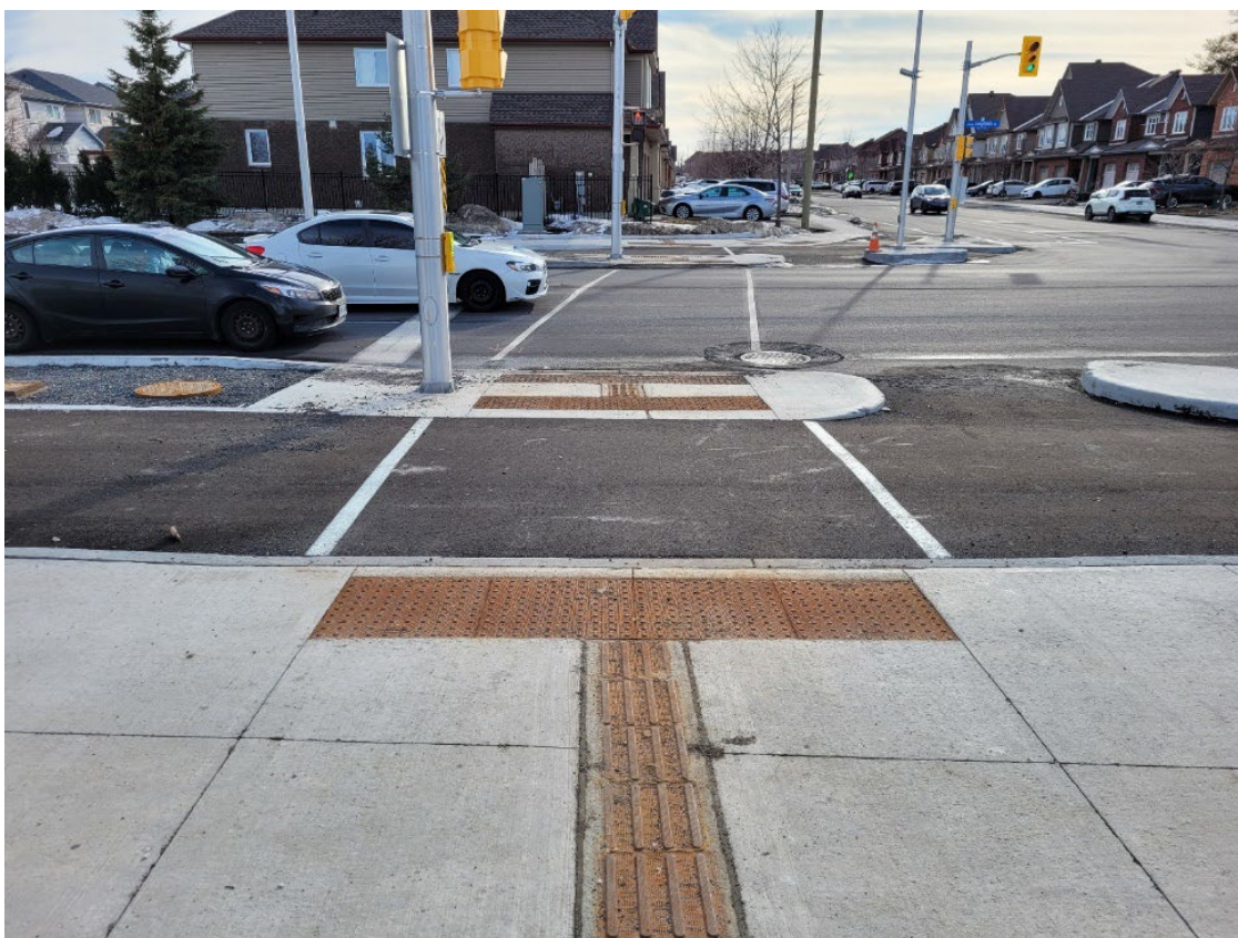
Figure 6.1: Tactile Features at a Protected Intersection
