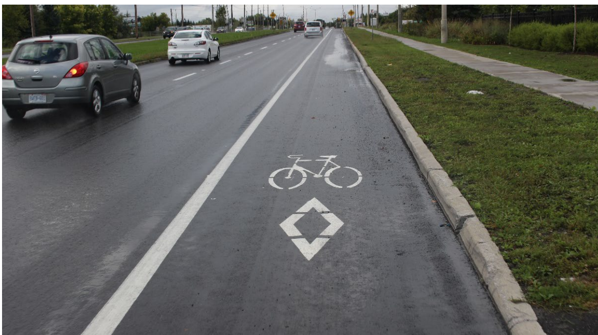
Figure 5.8: Conventional Bicycle Lane, Ottawa
