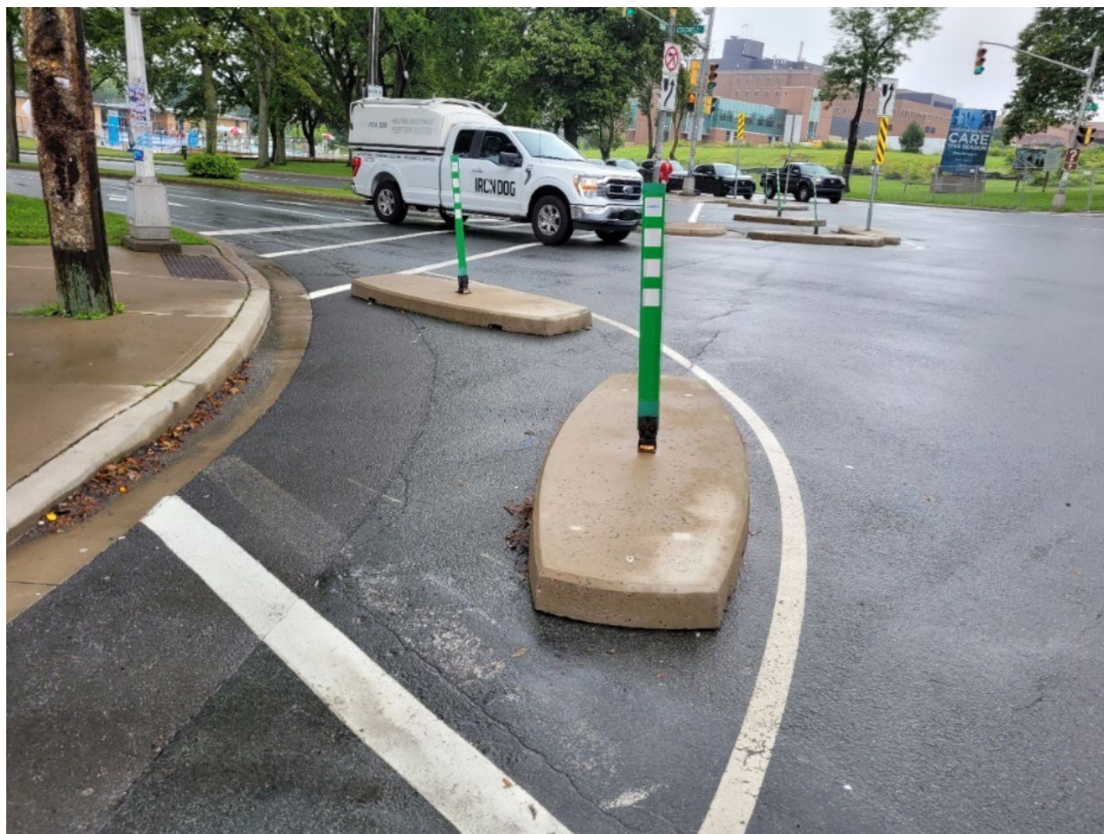
Figure 4.2: Turn Calming with Precast Concrete Islands, Halifax
