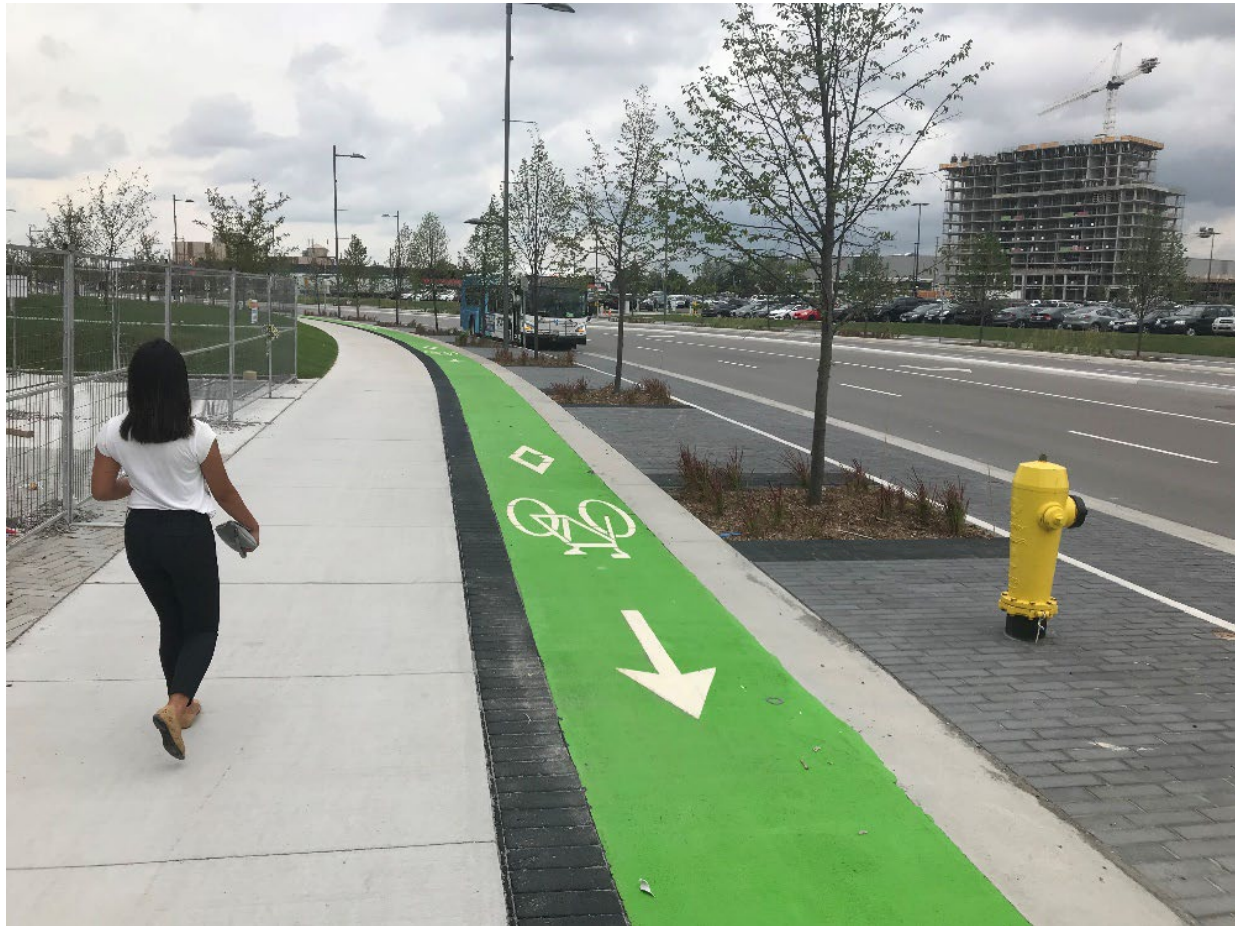
Figure 5.6: One-Way Cycle Track Separated From Sidewalk by Continuous Detectable Tactile Buffer Strip, Vaughan
