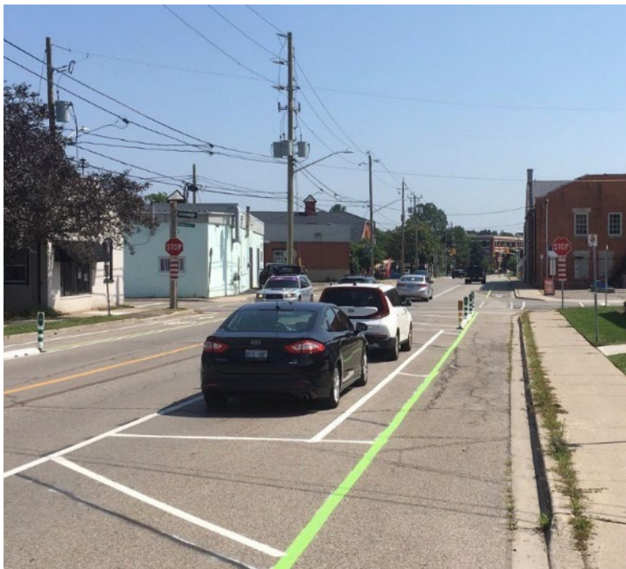
Figure 3.2: Parking Protected Bike Lane
