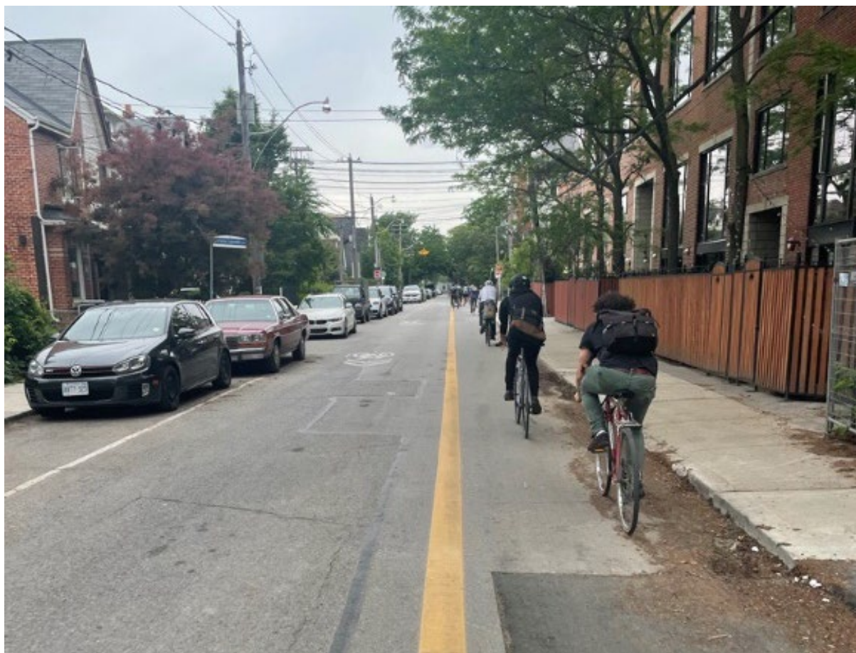
Figure 3.9: Contraflow Bike Lane
