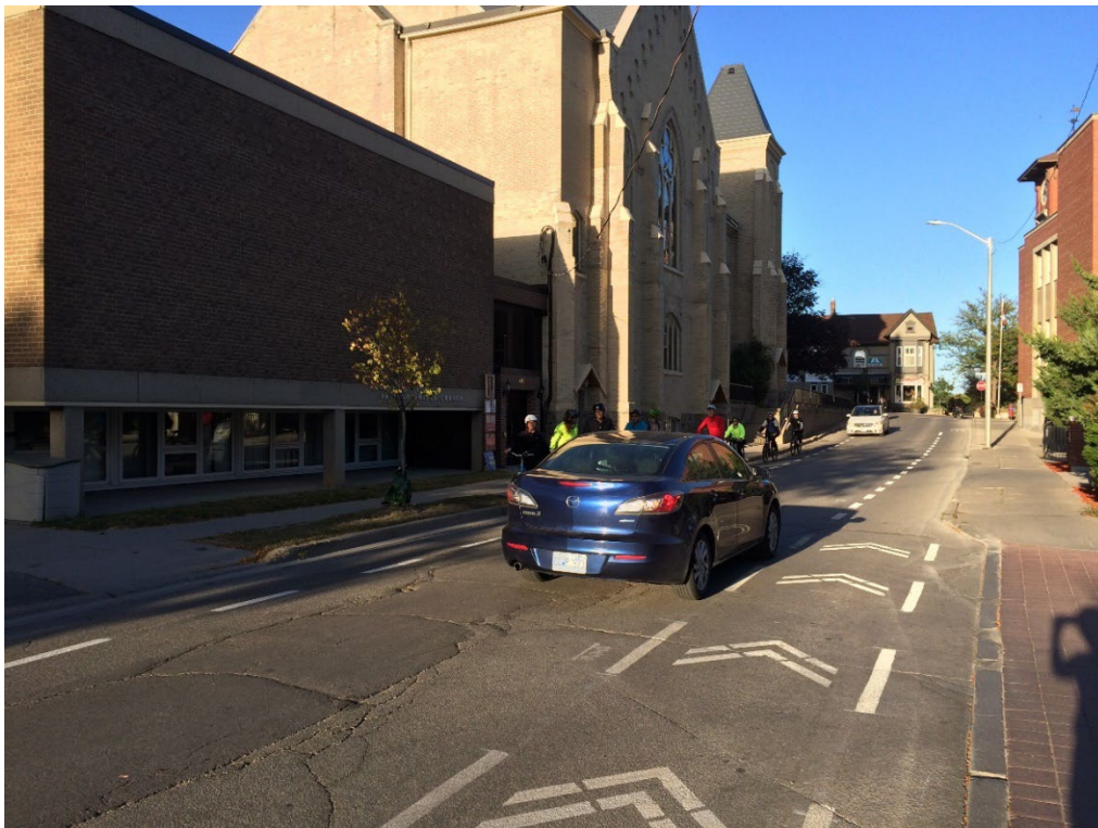
Figure 5.14: Advisory Bicycle Lane on Urban Street With No On-Street Parking, Newmarket
