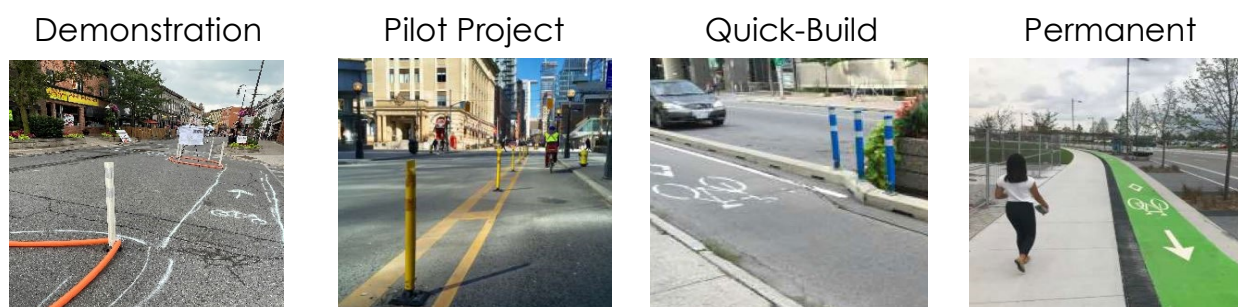
Figure 4.1: A typical example of the 4 stages of All Ages and Abilities facility development. The Rapid Implementation Network expedites the development process by going straight into the quick-build phase.
