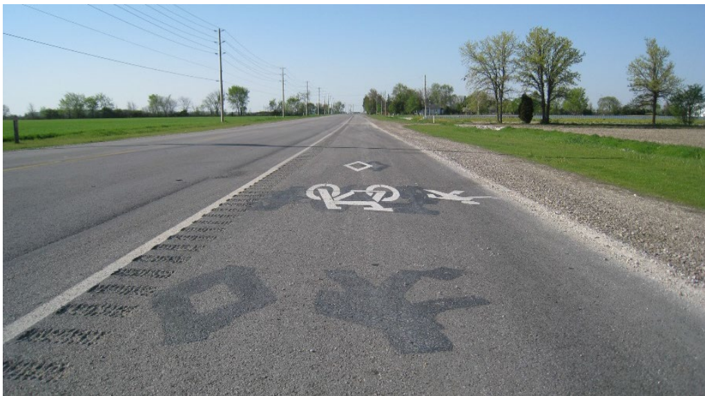
Figure 5.16: Rural Paved Shoulder With Rumble Strips, Essex County
