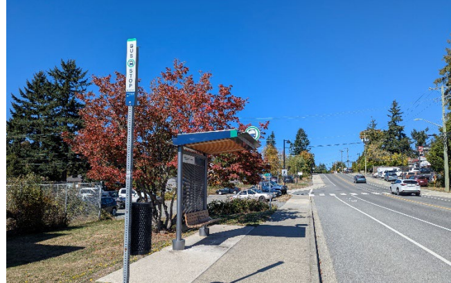
Upgraded transit stops and pedestrian pathways along Sooke Road improve accessibility and comfort for all travelers—supporting the community’s vision for safer, more connected streets.
