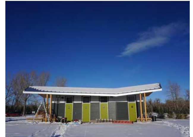
New Washroom Facility, Fish Creek Provincial Park, AB
