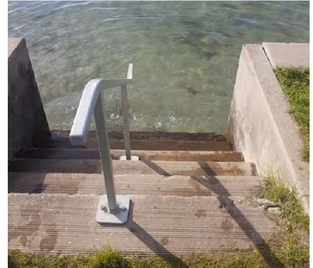
Stairs provide water access along Central Beach and Centennial Park
