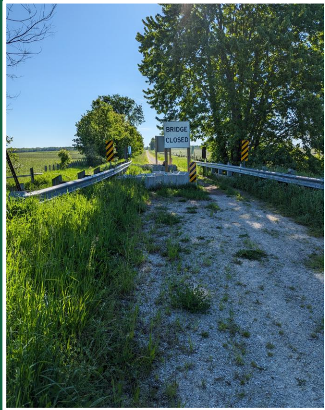
View of Structure Facing East
