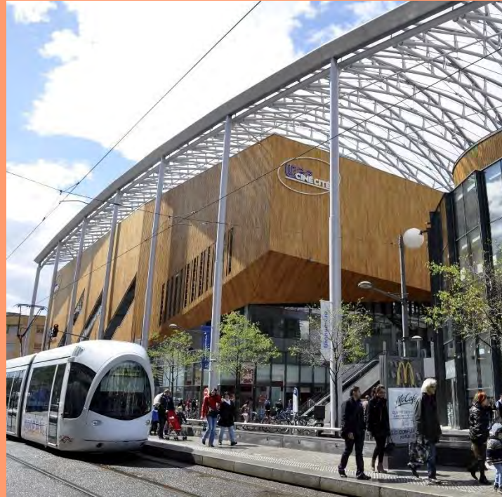
Photo 3.1p – Lyon, France (© Lyon Confluence)
