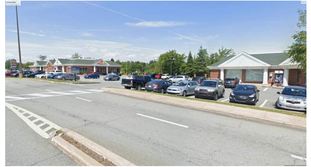
3. TOWARD EXISTING COMMERCIAL BUILDING
