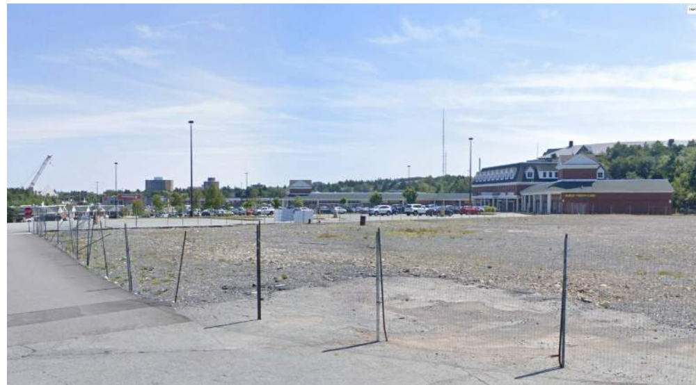
8. TOWARD DECOMMISSIONED CANADIAN TIRE SITE
