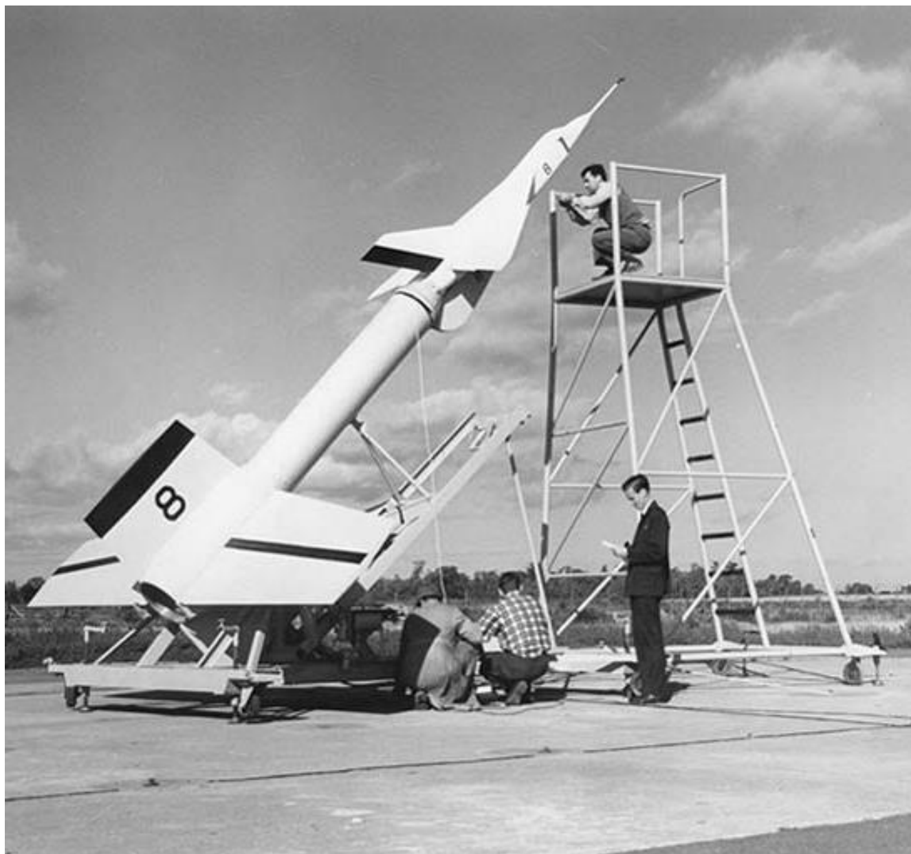
Plate 33: Avro technicians prepare an Avro Arrow test model attached to a Nike booster rocket to fire out over Lake Ontario at Point Petre in the 1950s. Retrieved from: The Orenda Ring | OTTAWA REWIND
