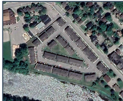
Townhouse Infill Development, Paris – 80 Willow Street (95 units)
