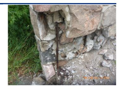
Details: OSIM bridge inspections identified components of the William Street bridge to be in poor condition or in need of rehabilitation work to meet current standards and practice. Items identified as high priority include the barrier system not meeting current Canadian Highway Bridge Code, no approach guiderails, poor condition sidewalks, inadequate sidewalk widths and lighting deficiencies.
