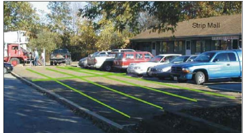
Figure 8.6. Communal Drainage Field Treatment System Located Under the Strip Mall Parking Lot (Joubert & Loomis, 2005).
