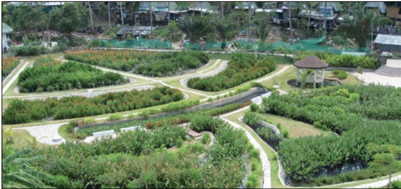
Figure 8.2. A Constructed Wetland in Ko Phi Phi, Thailand Treats 400,000 Litres of Wastewater Per Day from a Nearby Decentralized Sewer System while also Serving as a Popular Public Park (Austin, 2013).
