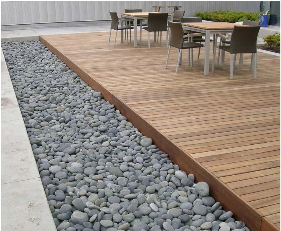
Northeast Office Building Rooftop
