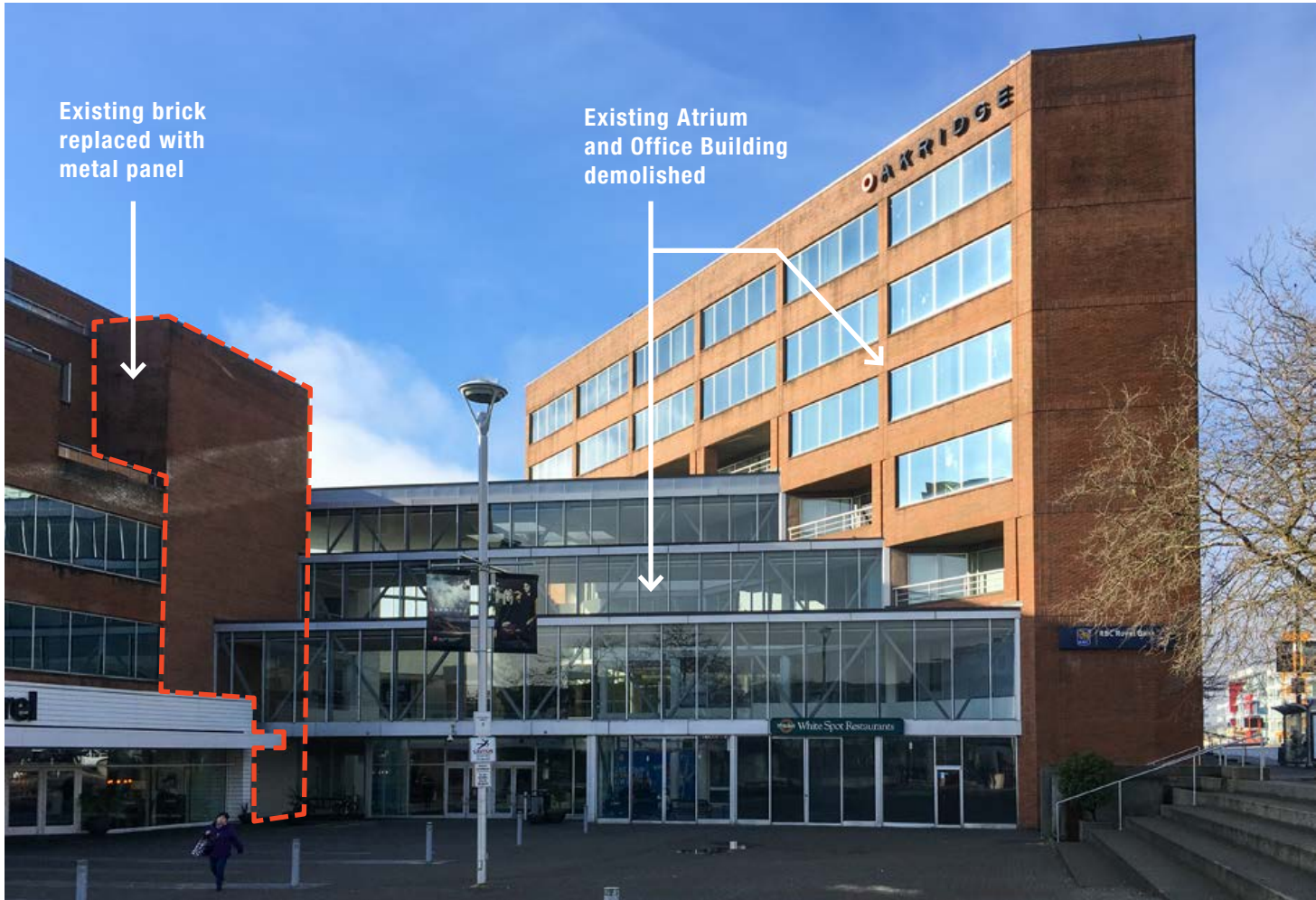
View of Northeast Office and Atrium
