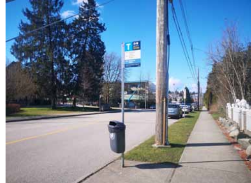
Existing sidewalks and bus loading zones on 6th St north of 8th Ave are narrow and existing boulevards have utility poles
