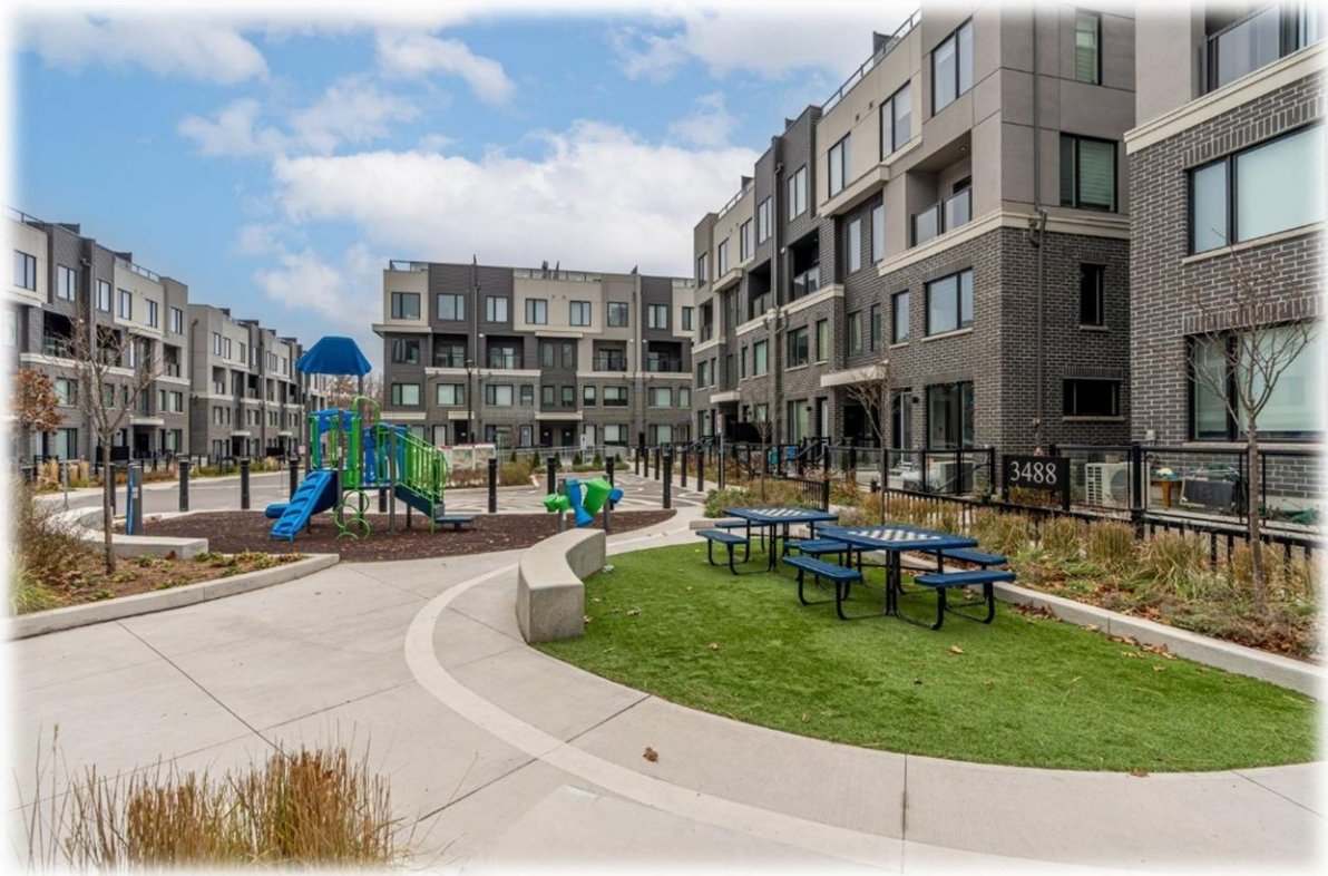
Figure 12: The Way Urban Towns, 4-storey stacked condominium Google Street View image. 4
