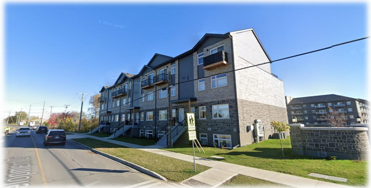
Figure 19: Creekside, 4-storey mid-rise apartment building Google Street View image. 10
