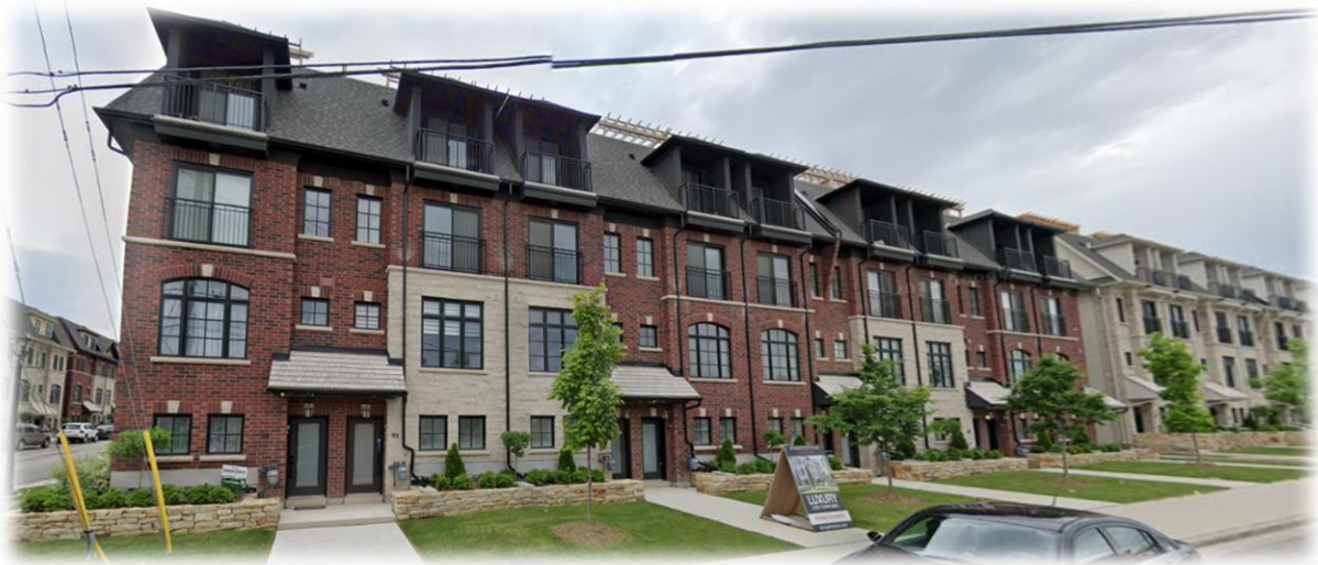
Figure 17: Streetsville Centre, 4-storey townhouse condominiums Google Street View image. 9
