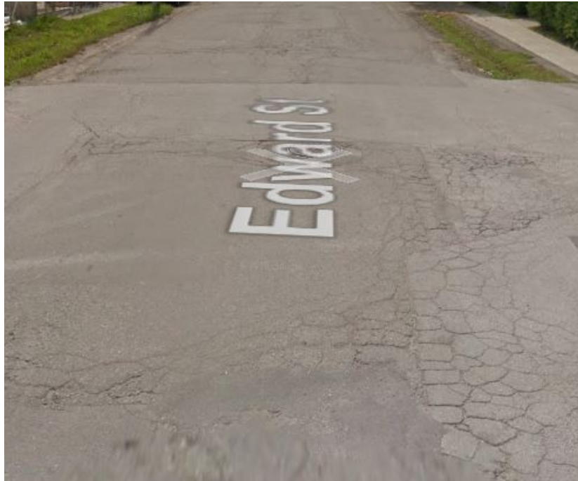
Figure 3: Cracking of Pavement
