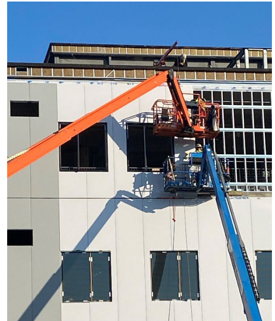
Workers install siding on the exterior of the new hospital.
