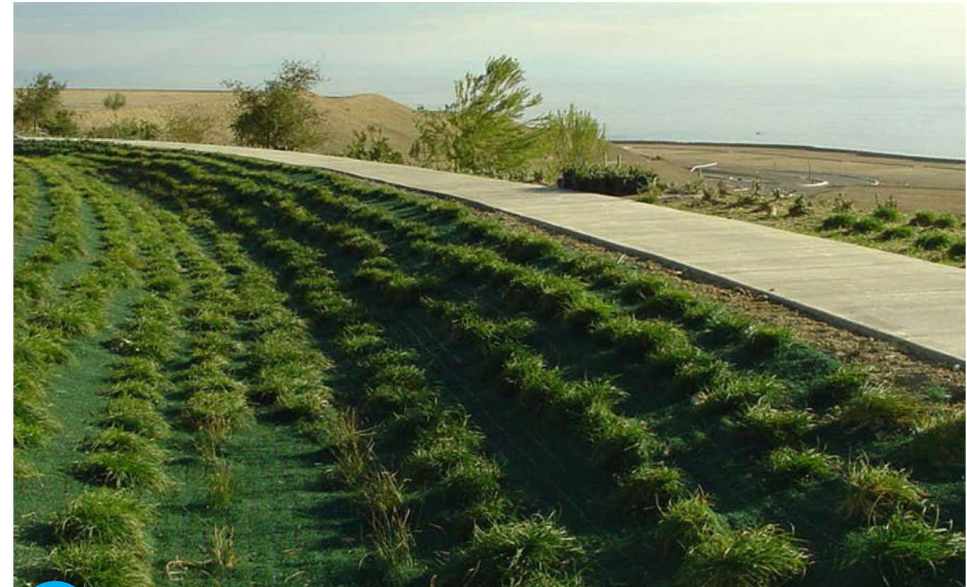
A Drainage swale next to waterfront promenade
