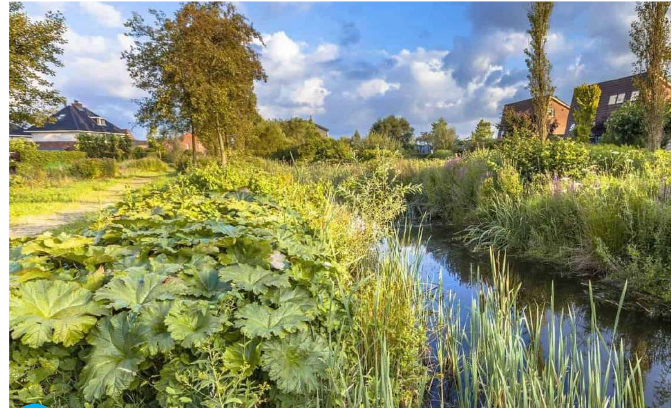
D Planted drainage swale
