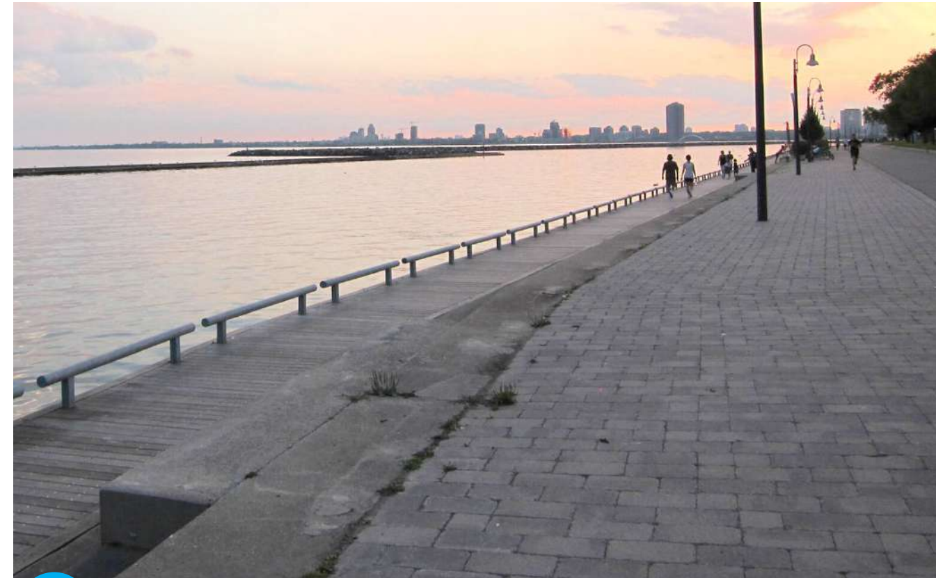
A Retaining wall with seating edge
