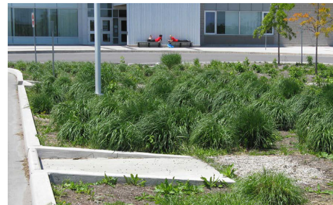
Image 4.35-4.37 Low-Impact Development practices at Markham's Bill Crothers Secondary School include bioretention areas, vegetated swales, constructed wetland type stormwater management facilities, and a rainwater harvesting system. Many streets within Markham Centre have good tree canopies.
