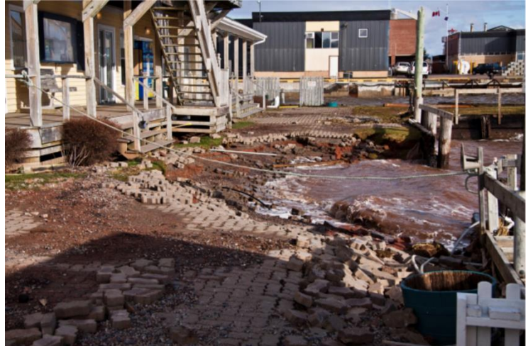
Figure 15: Charlottetown Yacht Club Storm Surge, December 6, 2010 (The City of Charlottetown, November 2024).
